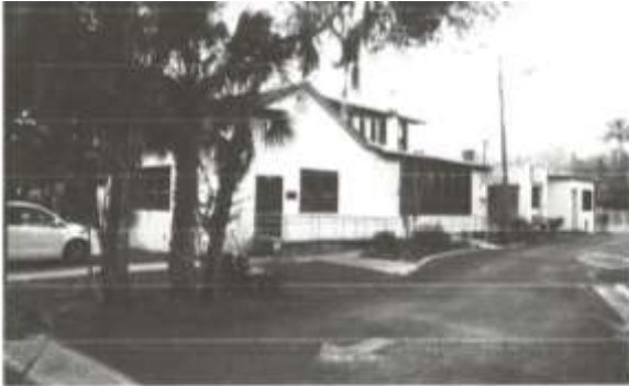
— Originally the Ormond Colored School, then renamed to the Rigby Elementary School, was relocated to 208 Central Avenue in 1924. It has been the PACE School for Girls – Volusia-Flagler since 1996. Source: Photograph by Randy Joyce (February 2021).
