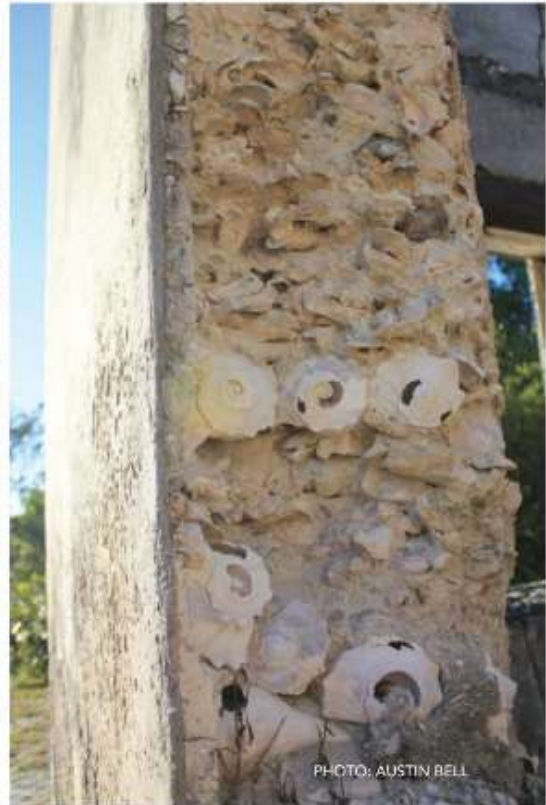
Top left: The John Foley Horr House sits on Horr Island, a 160-acre island in the Gulf of Mexico. Bottom left: Casey Wooster photographing Horr's Home Site. At right: The Horr House's tabby construction, a type of building material used in the coastal Southeast starting in the late 1500s, is part of what makes it unique.
