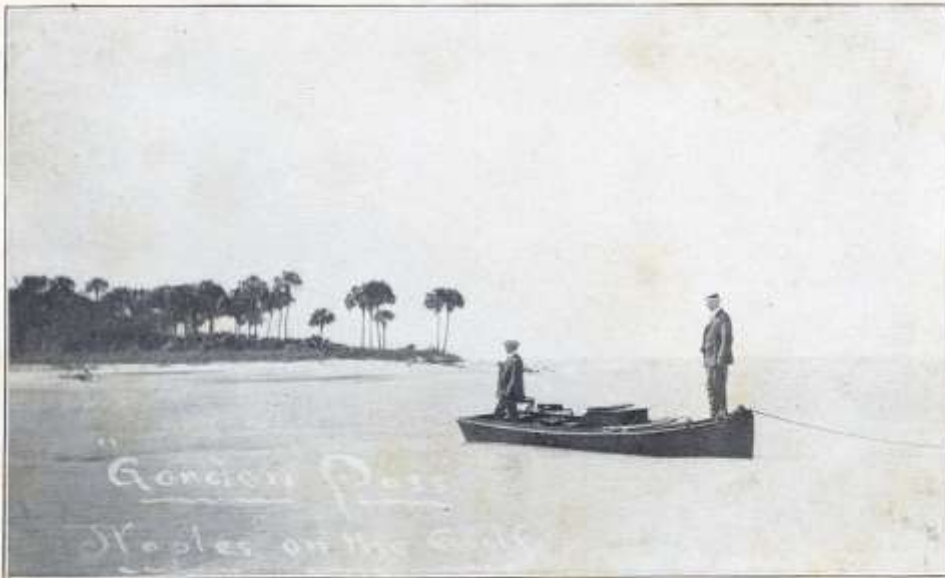
Gordon Pass—Entrance to Naples Bay, Naples, Florida.
